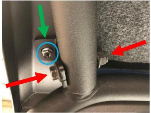
**Step (6)** Install the Upper Seal Plate on the unit by lining up the 10 center holes in the Upper Seal Plate with the 5 holes in the Front and Rear Roof locations as shown below. Then install the (10) 1/4" x 1" bolts with (10) 1/4" Seal Washers through the Upper Seal Plate and then through the Front and Rear Roofs.
